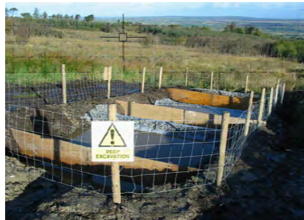
COMPLETED SETTLEMENT POND SYSTEM
